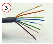
Position Wires into Correct Configuration (TIA 586-B Shown)
