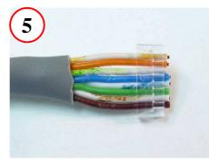
Insert Wires into –A192 Management Bar, maintaining alignment
