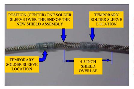
IMPORTANT: Fully clean and dry the first 5-6 inches of the existing harness shield. Use a cloth and Isopropyl Alcohol. Make sure that the first 5-6 inches of the shield is dry and has no unwanted material. This will make sure that there is a good electrical connection.
